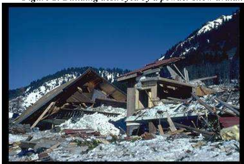
Figure 1: Building destroyed by a powder snow avalanche
